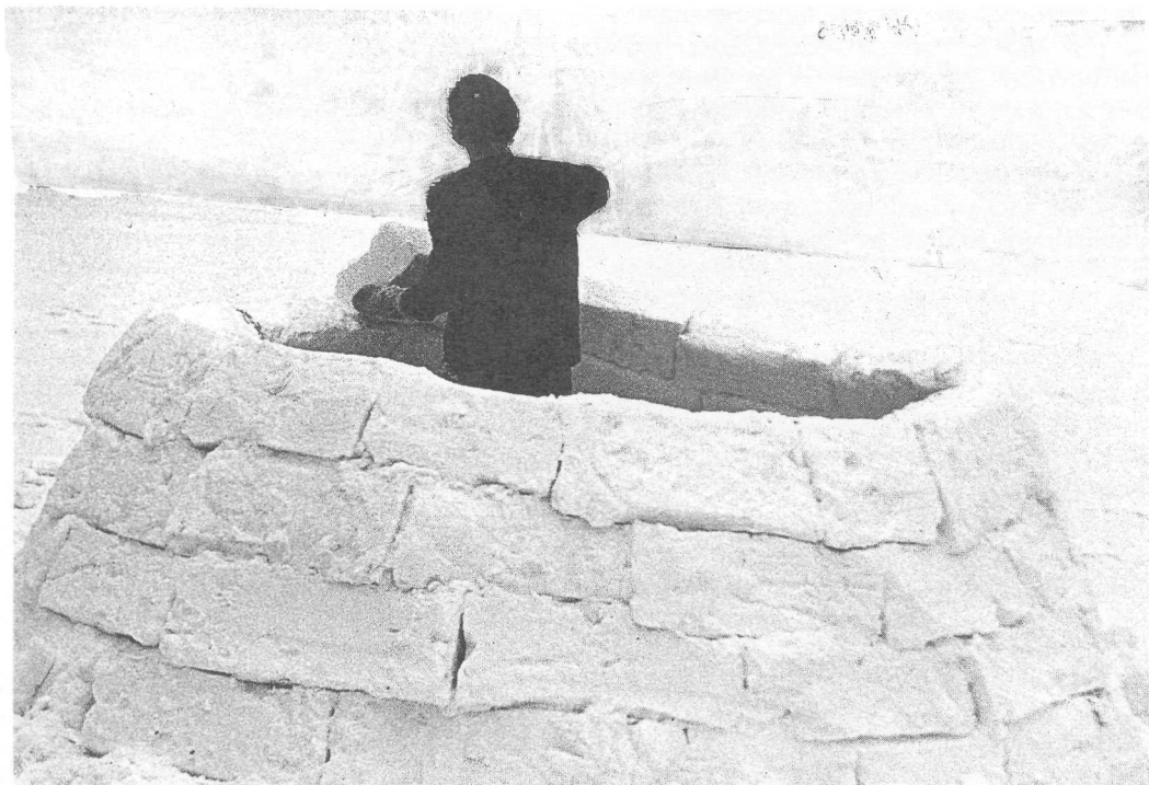
The secret to building an igloo is to use the force of gravity to lock the blocks together.
