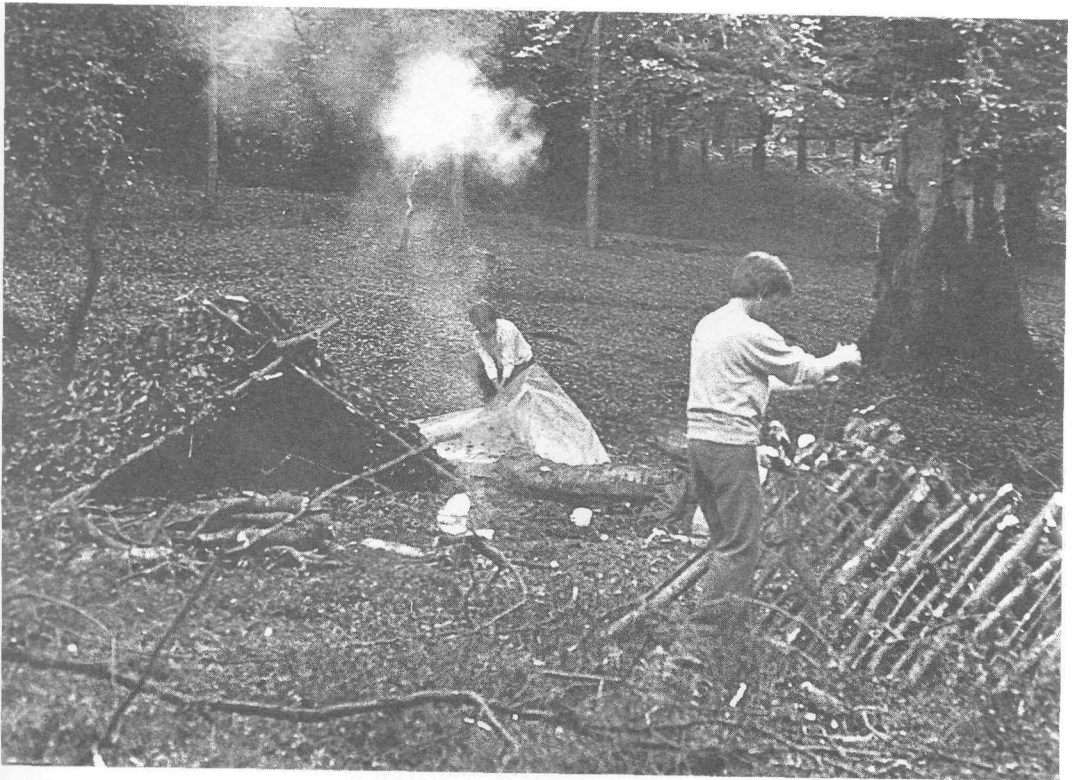
Large tipi-shaped shelters can be difficult to thatch adequately. By shortening two of the poles a one- or two-person shelter can be constructed. Because they are small they are strong and warm.
